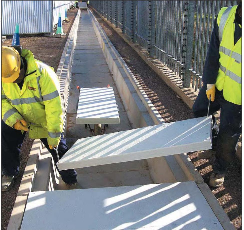
Installation process made easy through lightweight covers and lifting keys
