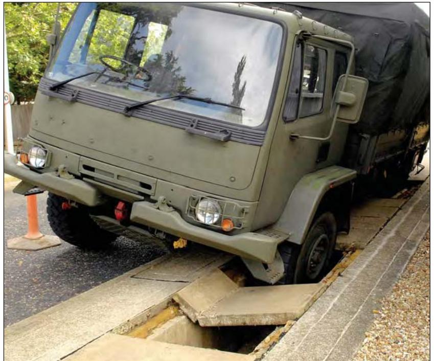
Damaged concrete trench covers in need of replacement to meet Health & Safety Regulations
