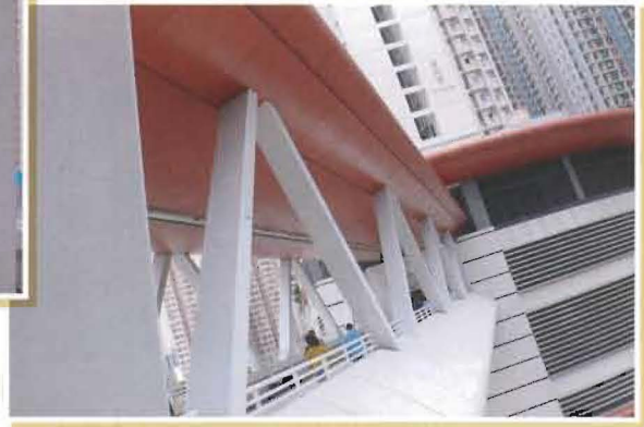
Footbridge Claddings at Yau Tong Redevelopment Phase 5 油塘重建第五期行人天橋覆面工程
