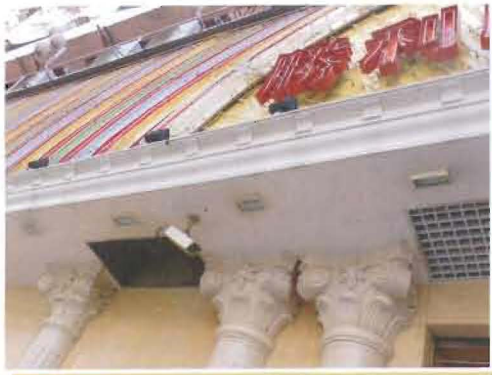
油麻地角線工程 Fiberglass Moulding at Yau Ma Tei
